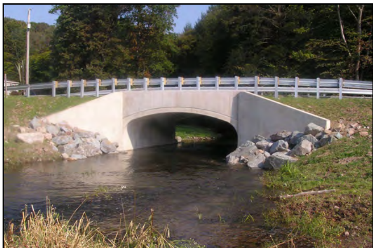
New Manchester Township bridge, owned and maintained by Wayne County
